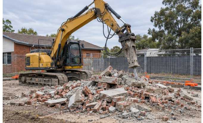
DEMOLITION AND STRIP-OUT
