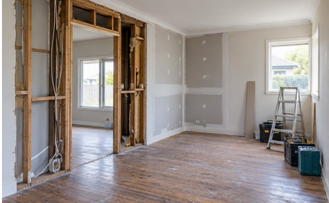
REPAIRS AND RENOVATIONS
